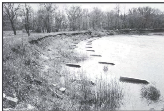
Wapsipinicon River bend at low flow, May 10, 1990, about two years after installation of Iowa Vanes.
