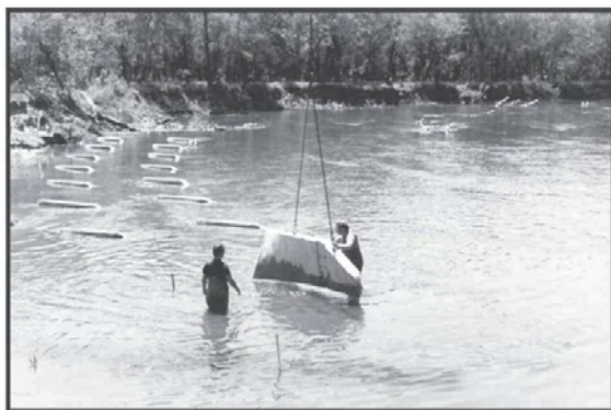
Installation of Iowa Vanes in Wapsipinicon River bend during low flow in the Summer of 1988.
